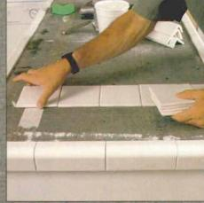
Layout starts from the center. To ensure a well-spaced layout, the author places whole tiles across the space, using a center mark as a reference. The remaining space is divided into two partial tiles.
