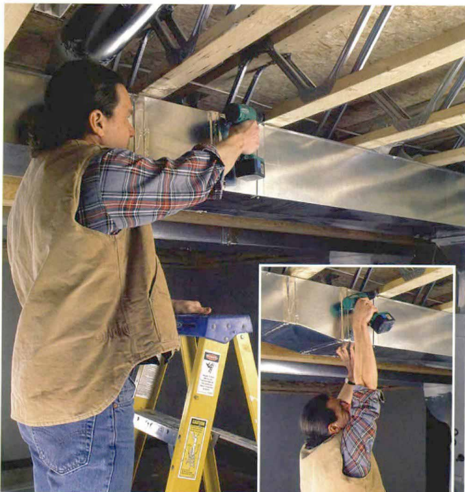
Wrist neutral (top photo) is the best working position. Flexing the wrist up or down (inset) while working increases the likelihood of developing carpal-tunnel syndrome.
