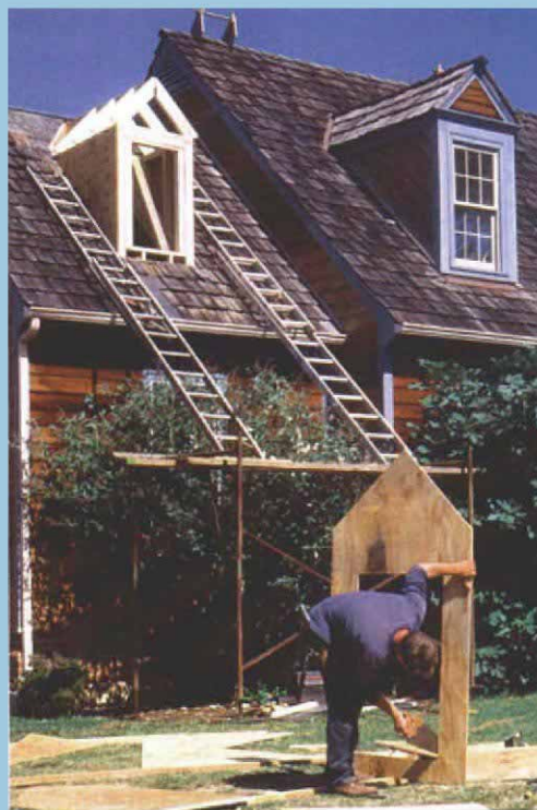
Spreading the load. A doubled-up 2x6 sits on top of the attic floor and spreads the load of the new dormer over four floor joists.
