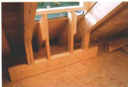
Spreading the load. A doubled-up 2x6 sits on top of the attic floor and spreads the load of the new dormer over four floor joists.
