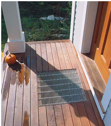
Details that ease New England winters. The main entry to the house faces south, so ice and snow melt off on sunny days. The floor grate allows snow stomped from boots to fall to the ground below. Photo taken at C on floor plan.
