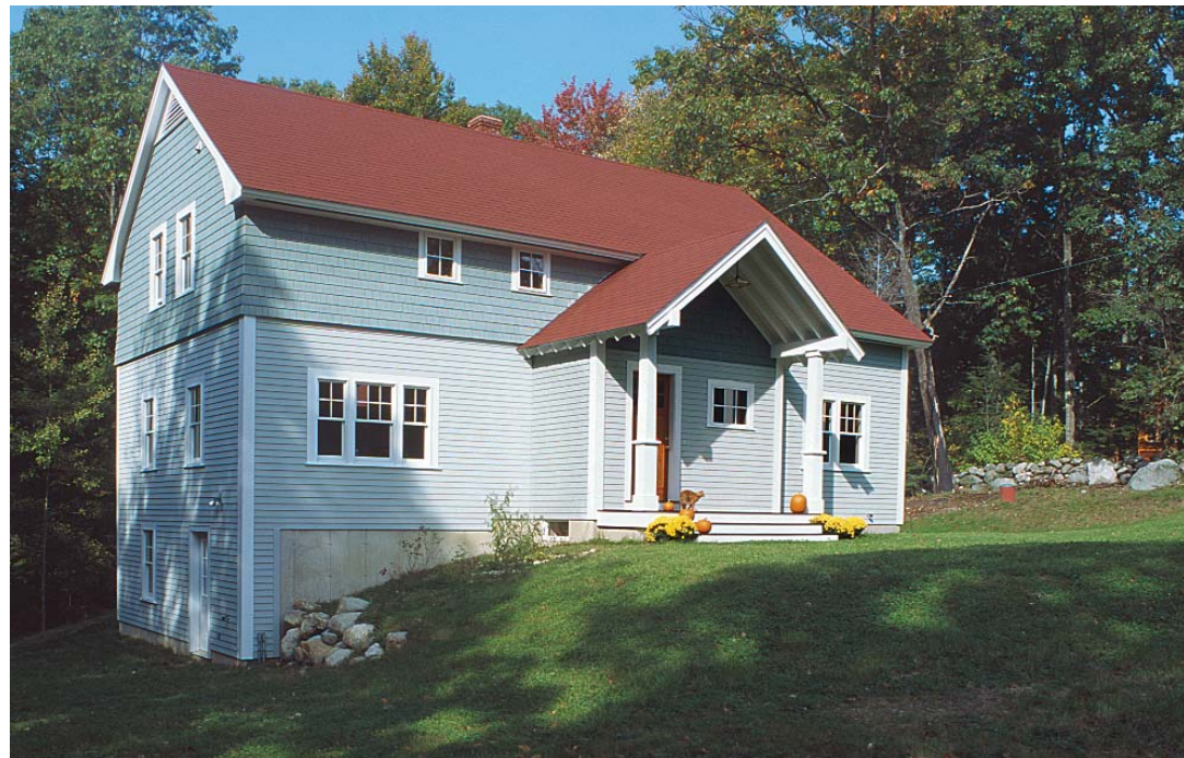
Porch does more than protect the entry. It also blends in the main roof as it extends over the bumped-out section of the first floor to the right of the front door. Photo taken at D on floor plan.
