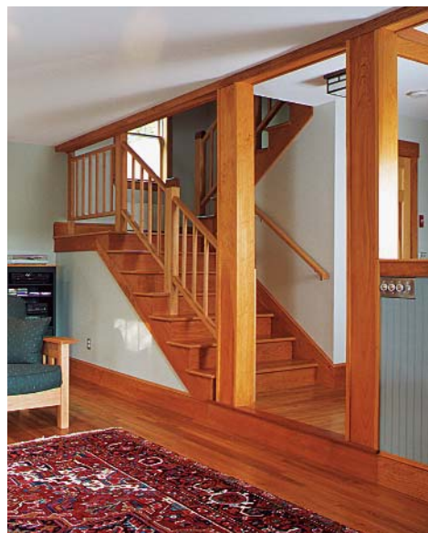
Most trim in the house is 4/4 pine. Where the edges of the boards show, heavier, more expensive 5/4 stock was used. Photo taken at F on floor plan.
