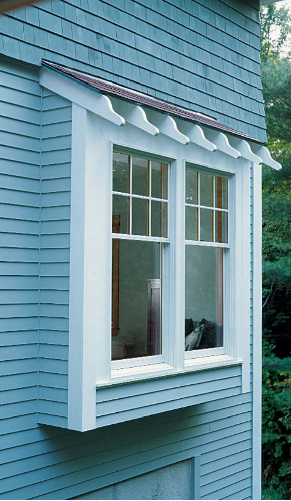
North-facing window seat gets even natural light for reading. Exposed rafter tails are a detail borrowed from older bungalow-style homes. Photo taken at B on floor plan.
