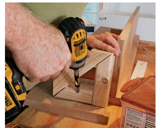
The first step is unique. Preassembling the first tread and riser allows blocking for the newels to be attached with hidden screws.
