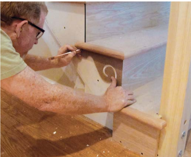
Attach the brackets. After mitering the brackets, mark them to length in place, then cut them and nail them on.
