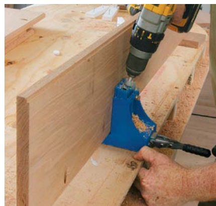
Drill pocket holes in the riser backs. Screws driven through these holes pull the risers tight to the treads, ensuring strong glue joints.
