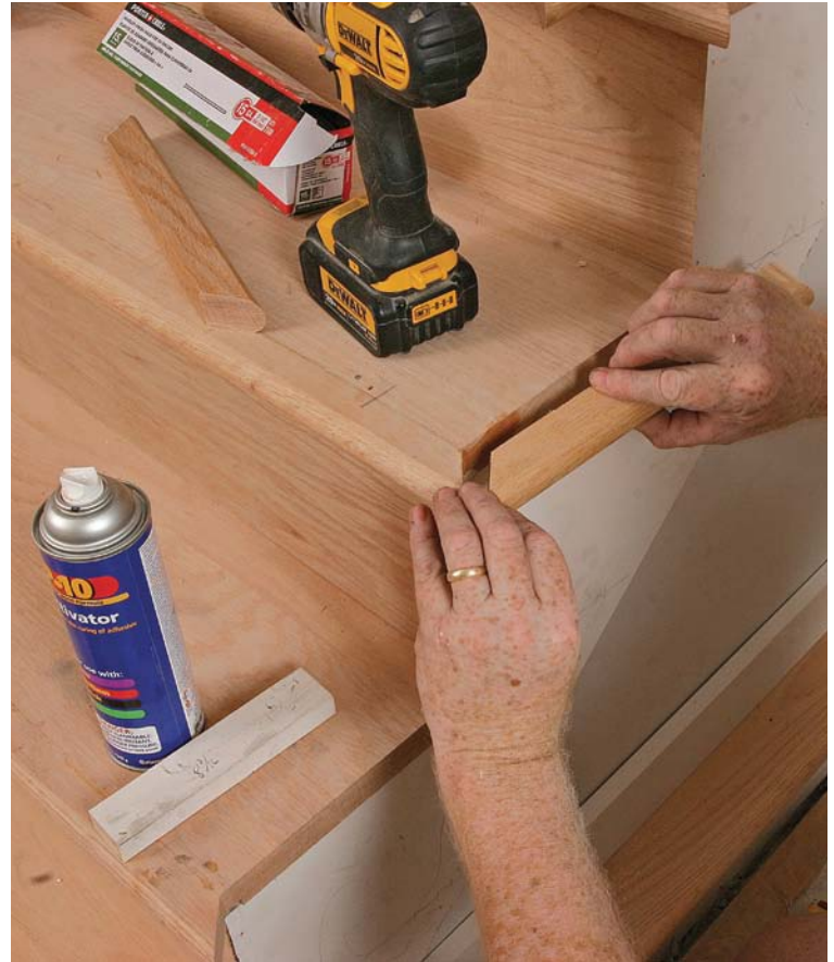
Use glue and nails. Glue each tread return at the miter, and join it to the back of the tread with 15-ga. trim nails. The glue holds the miter tight, and the nails allow the tread to expand and contract.
