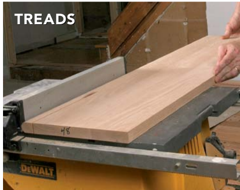
Rip the nosings off. Index marks made before cutting help to align the pieces for glue-up. Square-cut the treads to length, and miter the nosings.
