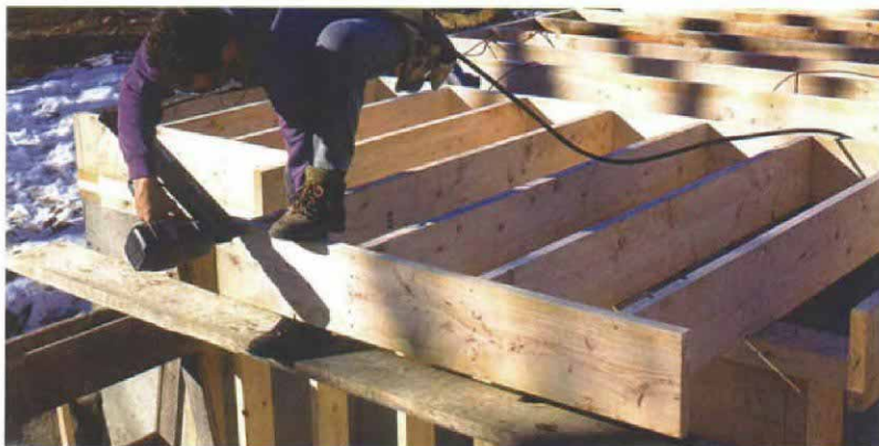
Outer rim joist is left long. Rim-joist stock is nailed to the cantilevered joists and left long until cutlines are transferred from the plates.
