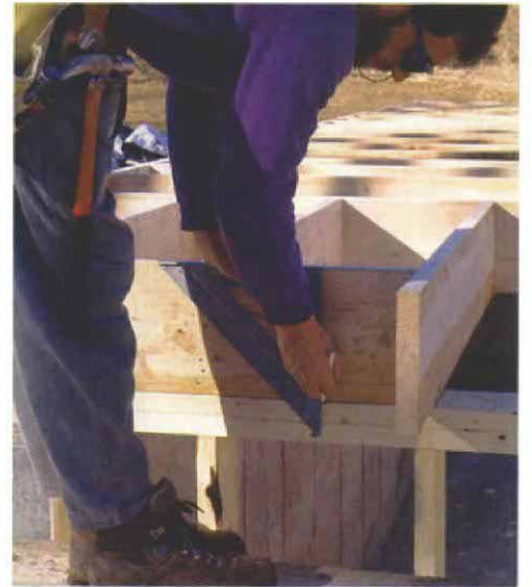
Bay joists hang off the main joist. When the bay joists run perpendicular, they are nailed to a main joist. After the cantilevered joists are attached, the main joist is tripled, and joist hangers are installed.
