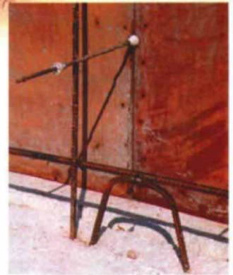
**U-shaped dowels replace keyways.** Planted on 4-ft. centers, the dowels help to anchor the footings to the walls and to the rebar.
