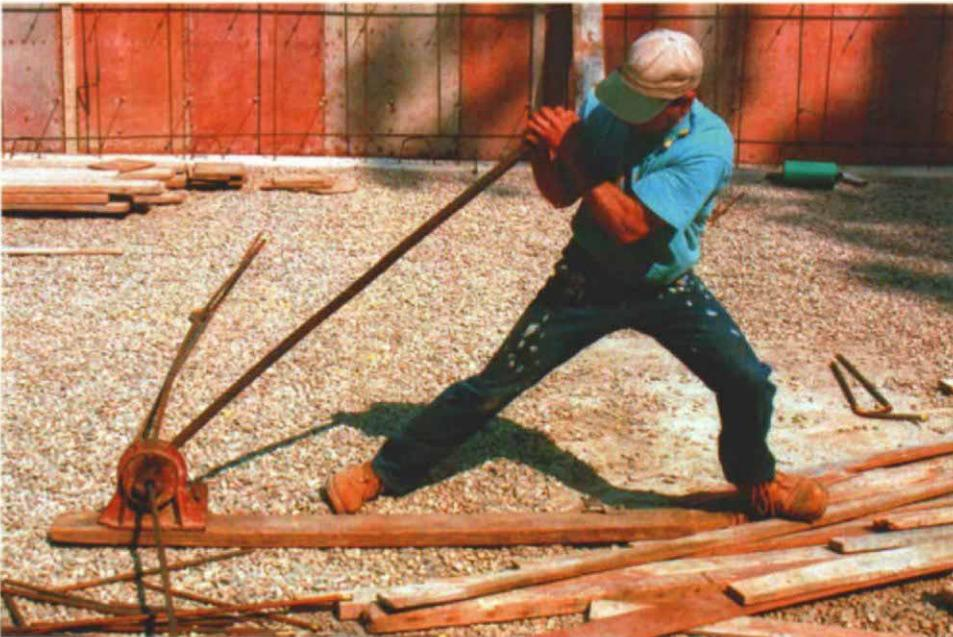
**Cutting and bending rebar is a matter of leverage and muscle.** Although chopsaws or torches can make quick work of cutting rebar, at a site without electricity, the stock can be cut with the cutter/bender (photo above). The tool's head provides a lever and fulcrum that makes simple bends as well (photo facing page); more complex bends can be made from individual pieces lapped together.
