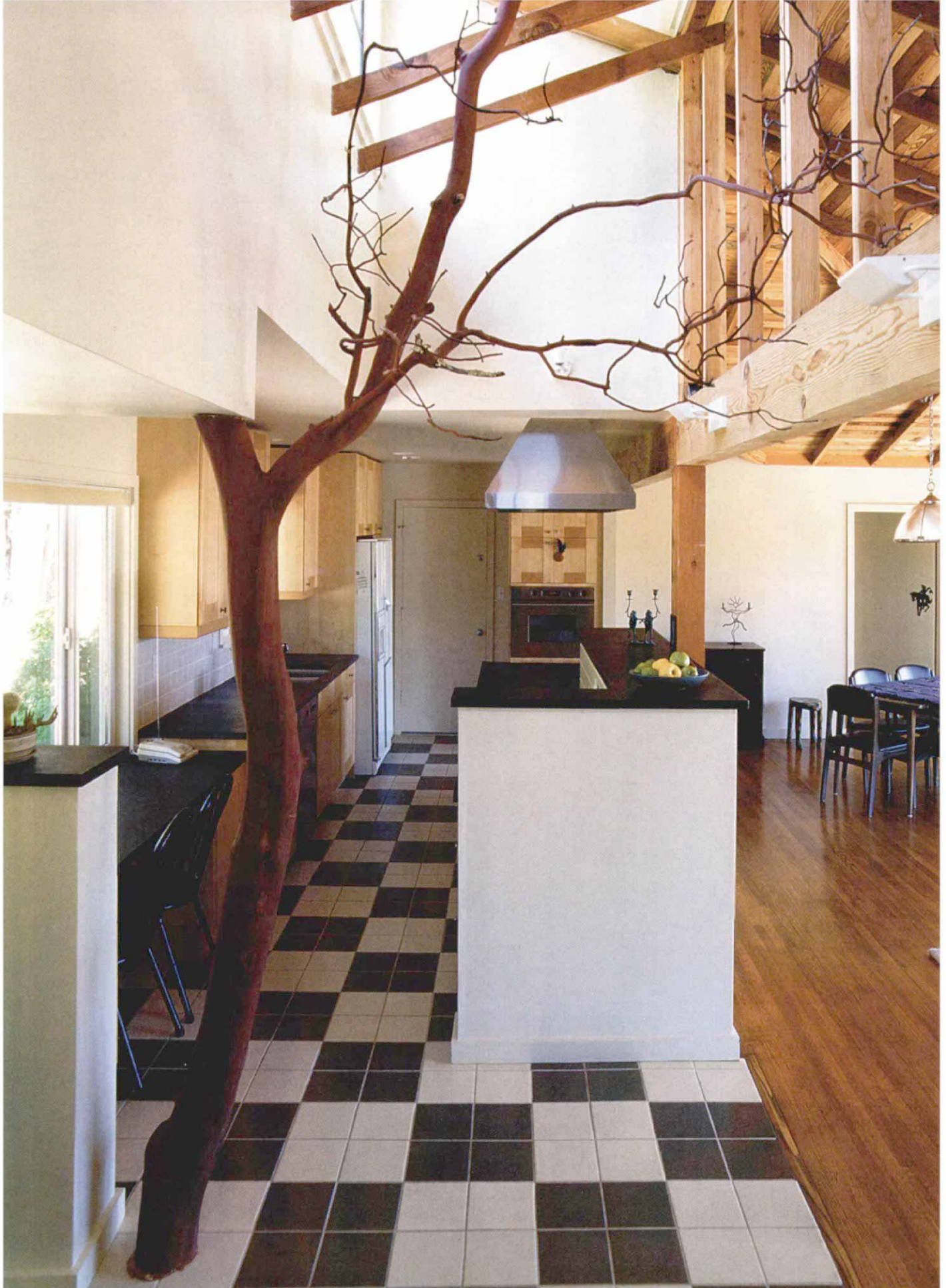
Bright, open space. While the cupola admits light, a beam replaces bearing walls that divided the kitchen from the living room. The madrona-tree column connects the interior space with the outside. The darker 2x4s are the old rafters. Photo taken at A on floor plan.
