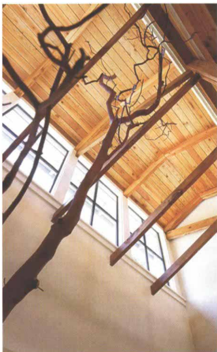
Reaching for the sky. Above the madrona tree, the cupola adds 62½ sq. ft. of glass to light the kitchen and great room. Overhangs limit intense summer sun but allow the winter sun to enter.
