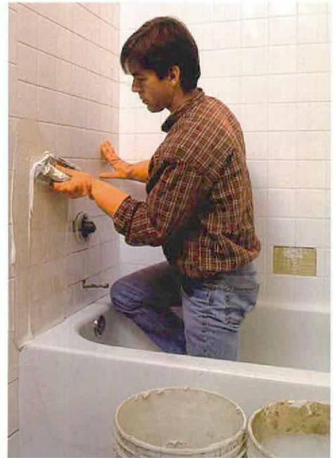
**Wall grout starts at the bottom.** To control the flow of grout, the author begins grouting low and works upward, packing the joints with a slightly angled float. As on the floor example, a strong diagonal pass cleans up the excess.
