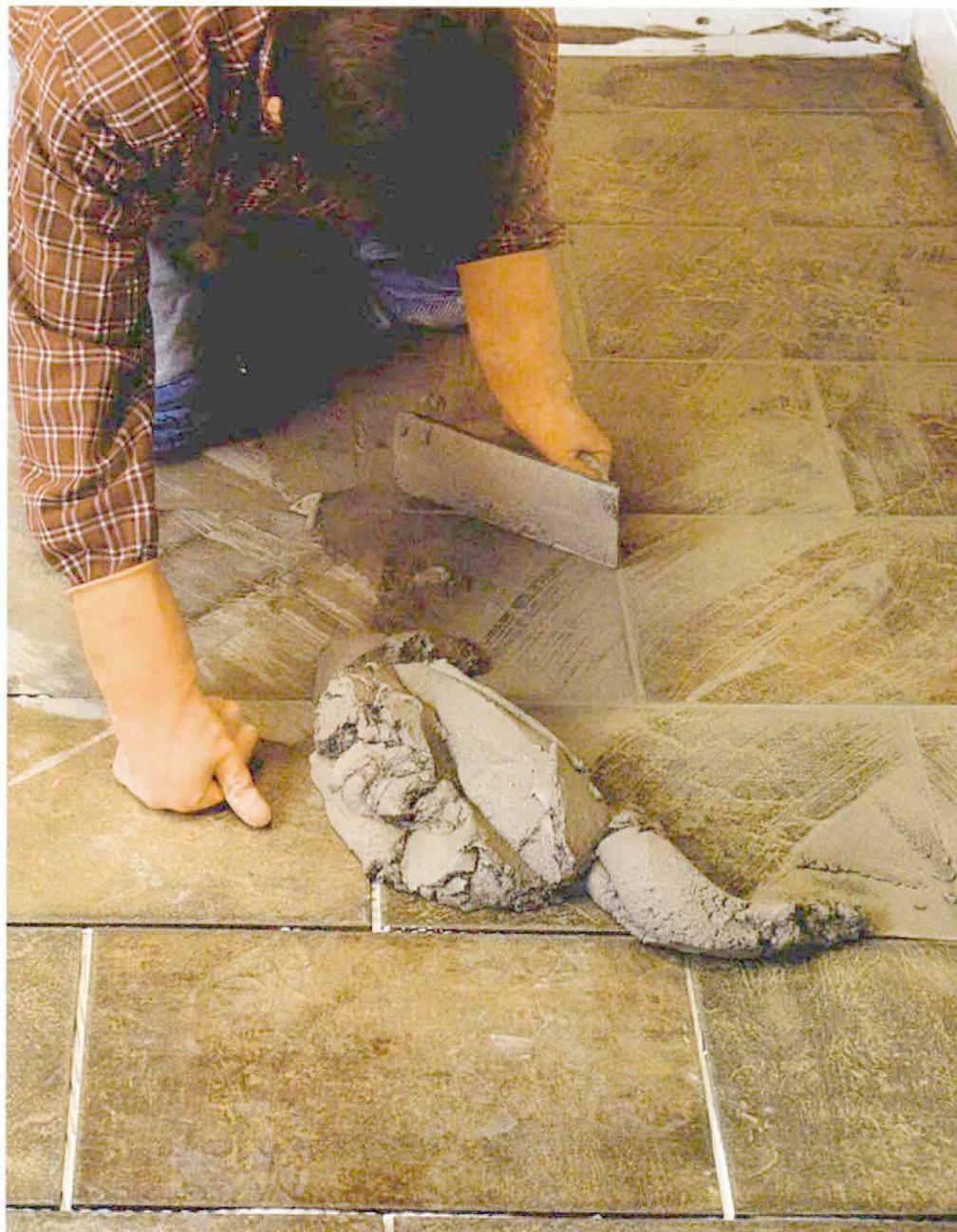
more than I can work with in that time. If I'm working in hot rooms or with porous tile, I spread just enough so that I can start the initial cleanup in 15 minutes to 30 minutes. I've also found that grout will set faster if left in the bucket, so I dump the entire mix onto the floor and keep it moving until it's gone.
