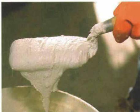
**Careful mixing controls the ratio of water to powder.** Mixing grout is often a process of estimating by eye; water should be added gradually to the powder to achieve the right mix. Clean water and a clean bucket are important ingredients.
