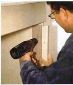
**Hanging doors starts with a drill press.** After testing the layout on scrap, the author drills 32mm holes in the backs of cabinet doors (above left). Pencil marks on the drill-press fence indicate the door-edge alignment. A jig locates screw holes for hinge plates inside the lower cabinets (above right).
