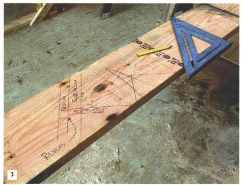
the rafter (calculations, p. 57). Next I set up a simple proportion using the roof pitch to find the rise dimension. Once I've determined the rise and run of the rafter, I use geometry to find the rafter length. Square the rise, square the run, add the two, and take the square root of the sum.
