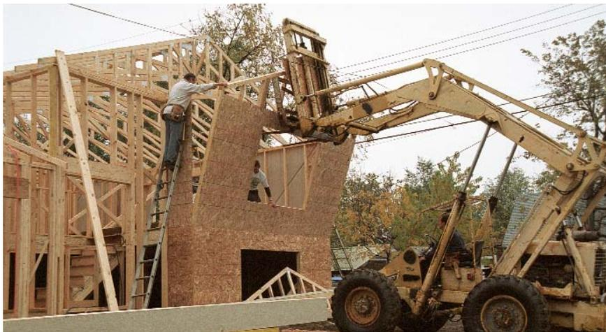
Leaving out the walls between kitchen, dining area and living area saves on framing and makes small spaces feel much larger (top photo). Using panelized walls enables a small, semiexperienced crew to assemble a quality house quickly (photo left). Savings on production costs make it possible to include luxuries such as skylights and vaulted ceilings.
