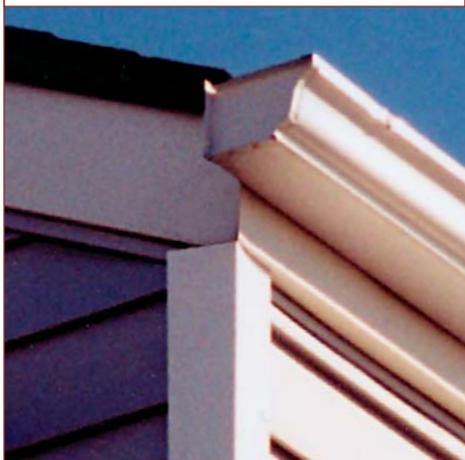
Even skilled framers get bogged down installing nailing blocks, lookouts and soffits on boxed eaves. These overhangs provide curb appeal, but a simple 2x6 fascia board with a gutter on it (photo above) provides an effective termination on less visible elevations. Scaling back the cornice work on these houses eliminated 60 sq. ft. of framing and cut down on roofing and painting, saving about \$250 without noticeably affecting the appearance.
