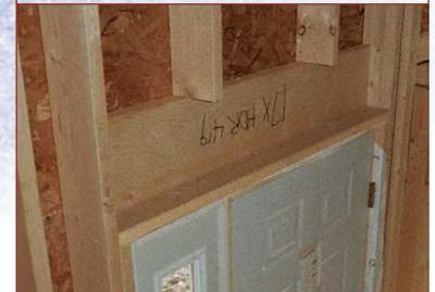
The standard practice of doubling up headers with a plywood sandwich in between wastes energy as well as material. A single 2x10 provides sufficient bearing capacity for most door and window openings. Adding a stud (on the flat) to the header's bottom edge creates a nailing surface and an insulation shelf.
