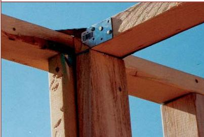
With careful planning, it's possible to eliminate a lot of superfluous framing material. Placing studs at 24 in. o. c., for example, saves nearly a third of the lumber consumed by a typical 16-in. o. c. layout. As much as possible, the author tries to eliminate double top plates. Single top plates (photo above) provide adequate structural support as long as the studs, floor joists and roof members are properly aligned to assure that the weight of each component bears directly on the one below.
