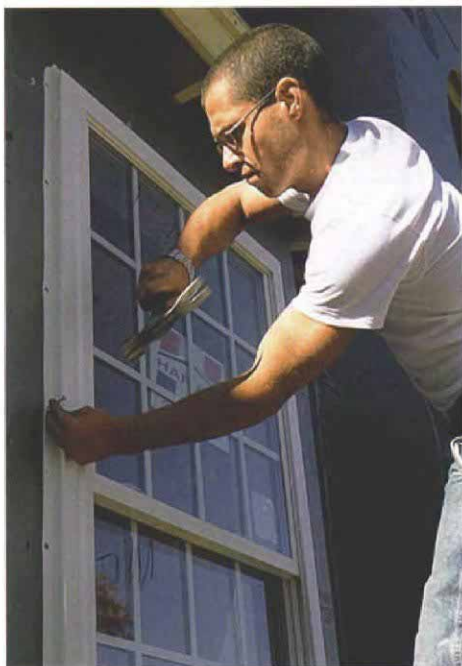
Plumb and square don't care what the material is. As the outside carpenter checks for plumb, the inside carpenter shims as directed.
