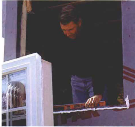
Installing vinyl is the same as installing other flanged windows. All window installations start with a level sill. One carpenter inside and another outside speed the task.
