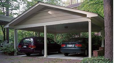
Why doesn't it blow down? It's easy to imagine a wind gust knocking over this structure that looks top heavy. Steel posts embedded in concrete and brick support the roof to stop that from happening.
