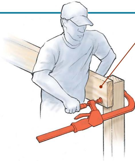
One hand positions a 2x10 against the post while the other tightens the clamp.
