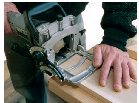
Before the casing leg is nailed in place, a biscuit slot is cut into the top.
