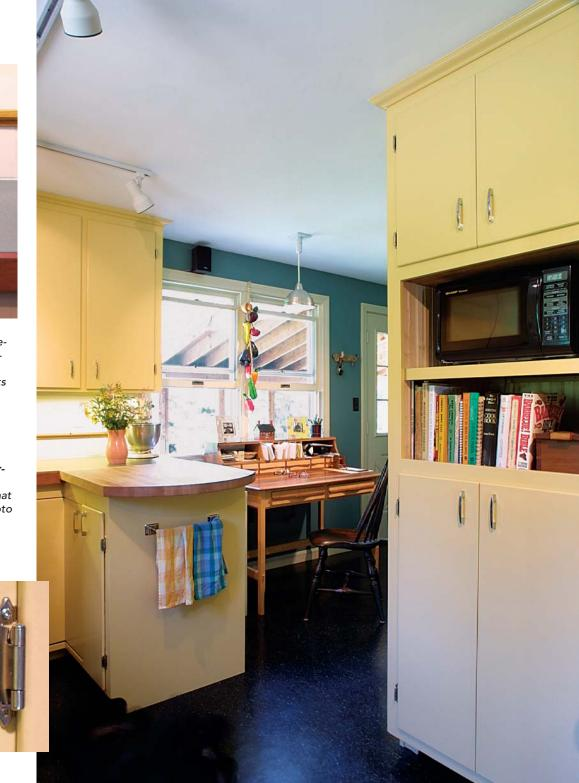
layer of <sup>3</sup>/-in. particleboard and glued down a new layer of laminate; this layering also raised the counter's height to a more comfortable level. The nosing is cherry (photo above left), glued and screwed to the edge of the substrate before the laminate is applied, then beveled with a bearing-guided router bit.
