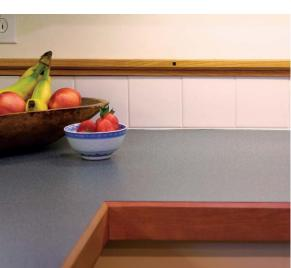
Hardwood nosing dresses up an inexpensive counter. To raise the level of detail on the new laminate counter, the author added a beveled cherry nosing. A smaller rail above the backsplash accents the plain white tile. Photo taken at B on floor plan.
