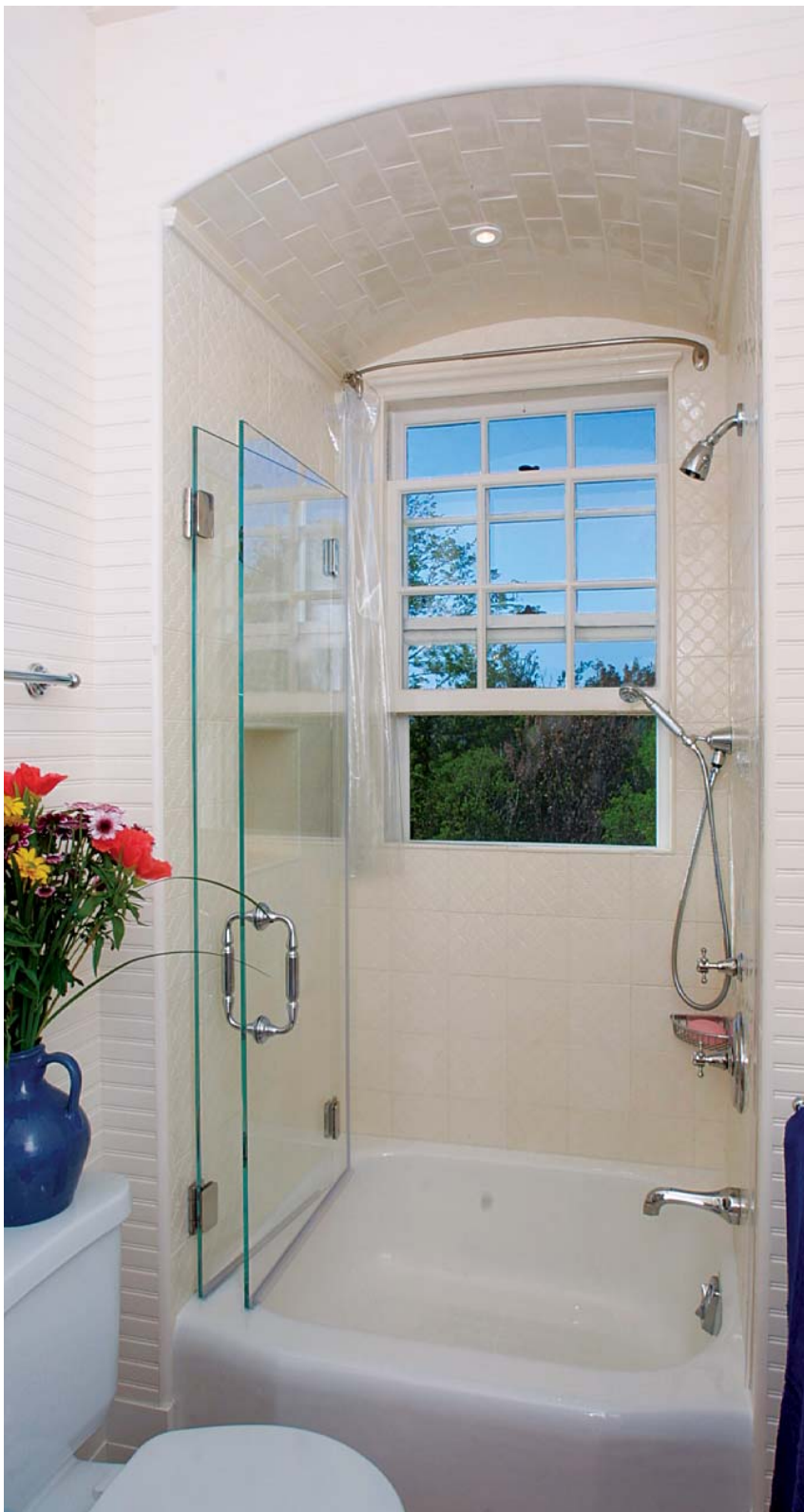
CHILD'S BATH: Barrel-vault shower. In a space only 42 in. wide, this tiled shower makes room for getting in and out by way of a frameless glass door that is hinged in the middle. The double-hung window has its own shower curtain to protect it from the indoor weather.
