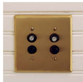
Don't forget the switches. Reproduction push-button switches are another finishing touch that shows attention to detail. Note how the cover plate just fits between the panel beading. It's no accident.
