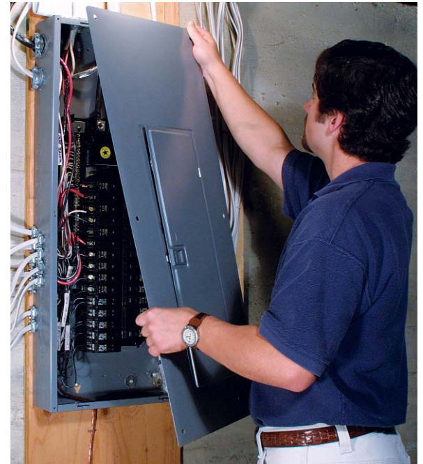
1 and 2. After locating the correct circuit, turn off power to the main breaker, then remove the service-panel cover.
