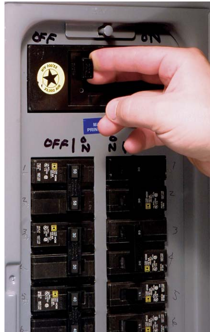
1 and 2. After locating the correct circuit, turn off power to the main breaker, then remove the service-panel cover.
