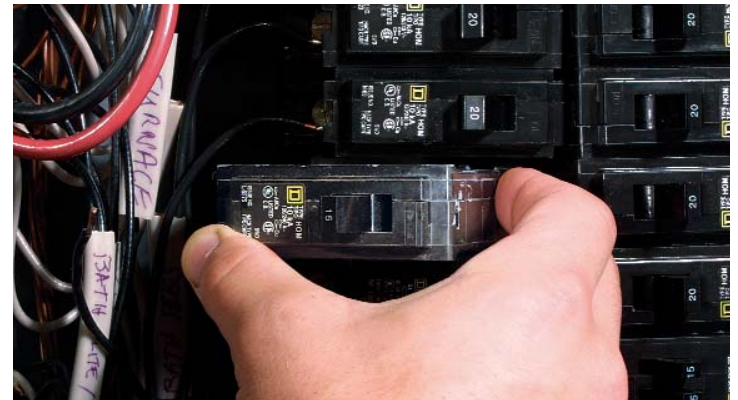
4. Remove the existing breaker from the service panel.
