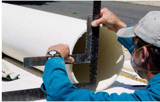
**Measuring the column in four places.** By marking four compass points on the column, it's easier to plumb the columns and to transfer the height measurements, which vary because the floor pitches.
