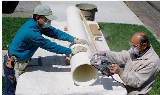
**Cutting the base.** With the height marked at four points, the base of the column can be cut with a circular saw to match the floor's pitch.
