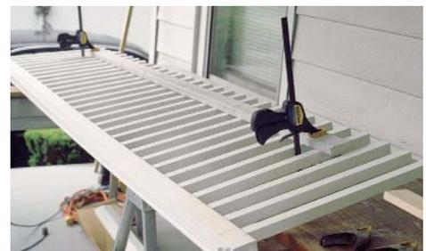
By clamping a wood strip to both sides of the balusters, the author was able to pick up and place this now-rigid section of railing without it racking or swaying.
