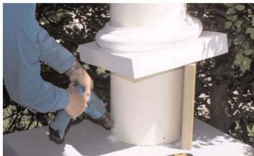
**Structural element with a finishing touch.** With the base lifted out of the way, pilot holes are drilled into the column. The column is secured with galvanized screws. The base slides into place, covering the screw holes.
