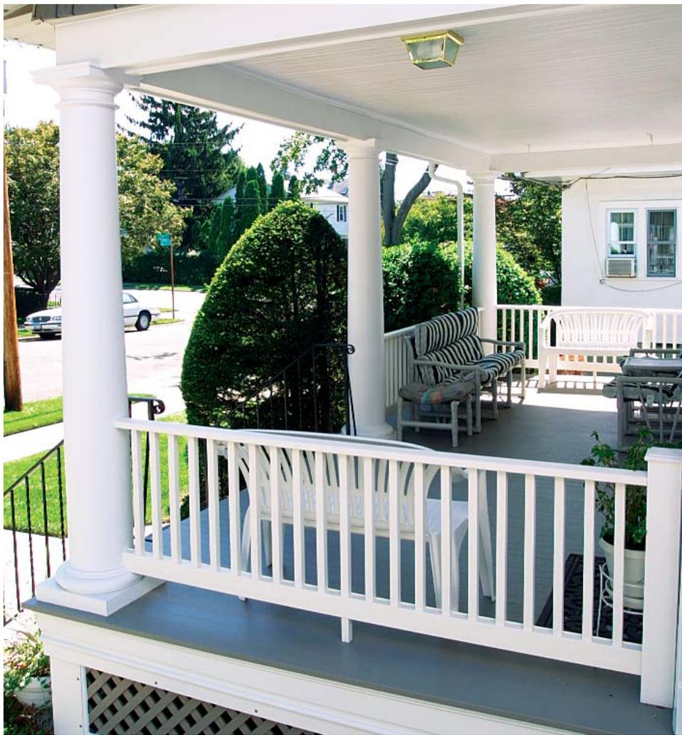
**Preserving a traditional look with PVC.** Reinforced polymer-composite columns and PVC railings make for a maintenance-free, architecturally correct restoration.
