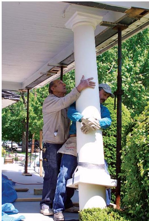
**Wrestling the column into place.** It takes two to place the column, but positioning it is easy by aligning the four points of the column to those on the deck. Note that the base is duct-taped out of the way.
