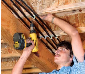
Clips support horizontal runs. To keep the tubing in place, plastic or metal clips must be secured every 32 in., or closer for straight exposed runs. It's important that the clips don't constrict or crush the tubing.
