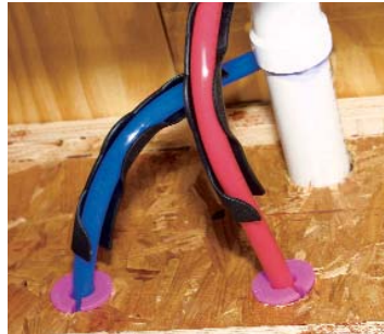
Plastic elbows support tighter bends. Tubing bent to a tighter than recommended radius or bent adjacent to a wall or floor penetration can be supported with plastic pipe supports.
