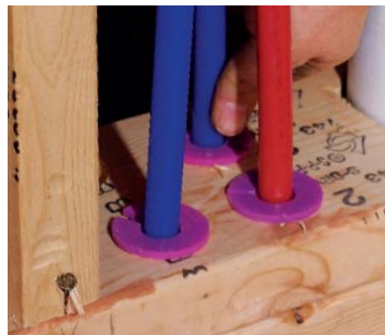
Nylon grommets protect the tubing. Available from most distributors, grommets are cheap insurance for tubing that passes through sharp-edged steel or wood studs.
