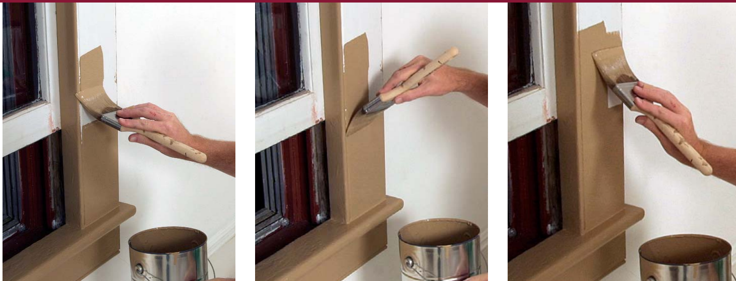
Paint back to make it blend. To ensure consistent coverage, the author applies paint in a back-and-forth motion (photos above left). To eliminate visible overlaps (such as brush strokes), he always paints back into the previously painted section (photo above right) before moving on to the next one.
