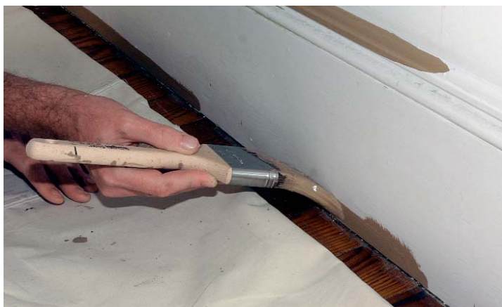
Fill in as you go. For maximum efficiency, the author applies paint in 3-ft. sections. When painting a baseboard, he cuts in the top and bottom sections using a lightly loaded brush (photo above left). Then he fully loads the brush and fills in the middle (photo above right).
