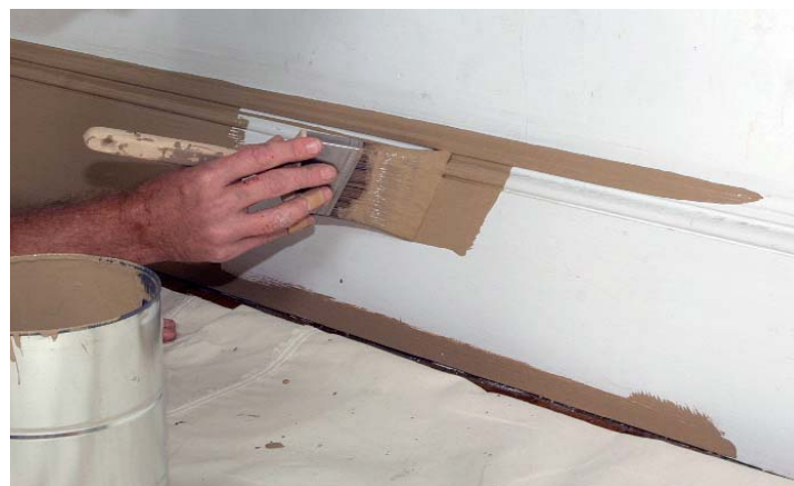
Fill in as you go. For maximum efficiency, the author applies paint in 3-ft. sections. When painting a baseboard, he cuts in the top and bottom sections using a lightly loaded brush (photo above left). Then he fully loads the brush and fills in the middle (photo above right).
