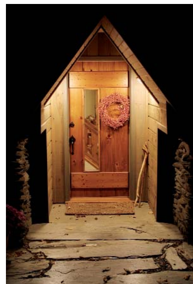
A welcome sight on a stormy night. The well-lighted front door is protected from the elements under a dormer carved into the deep eave. The door’s plywood core is sandwiched with 5/4 white pine and varnished to an antique patina, making it both inviting and stable. Photo taken at I on floor plan.
