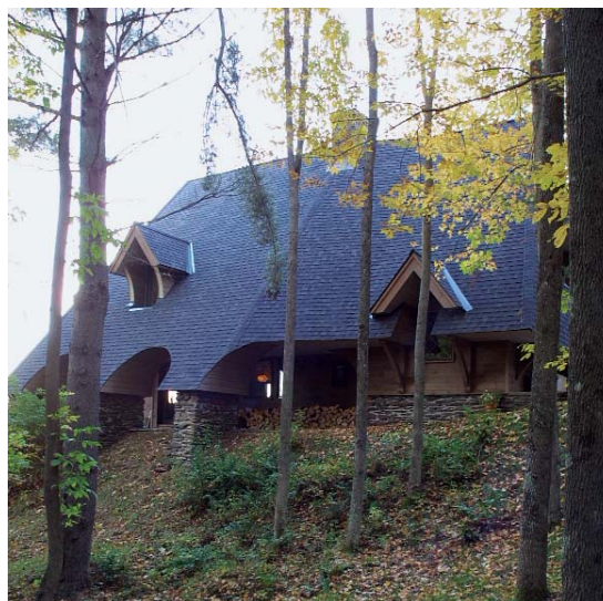
Under the big top. The steeply pitched roof extends over the native-stone terraces, giving this 1600-sq. ft. cottage a massive first impression while protecting it from Vermont's fierce winters. Photos taken at A, B and C on floor plan.
