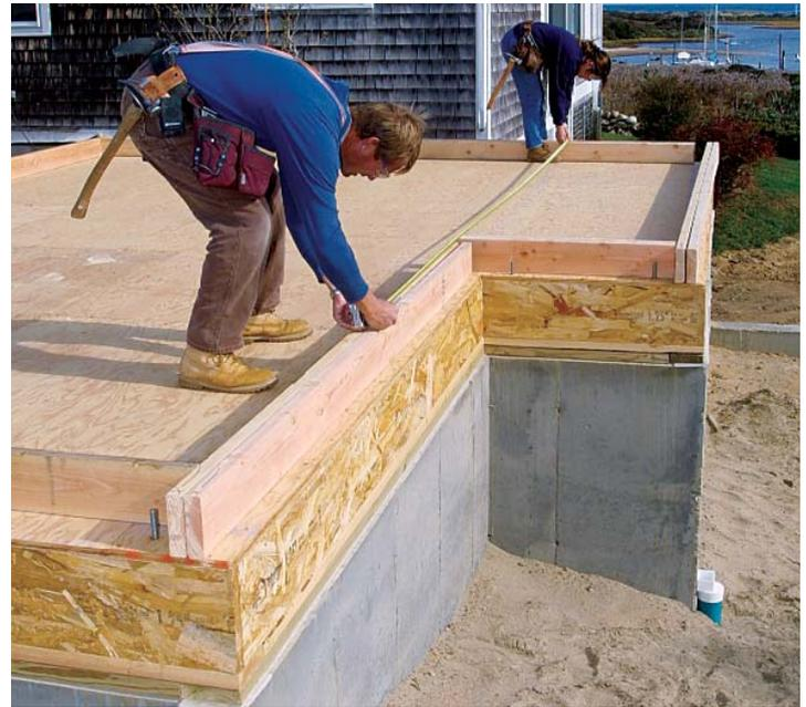
bers) for the exterior walls (top photo above). In this step of layout, we set the plates side by side on the layout line, and every wall-framing member is located and labeled. With this information, we assemble the walls on the floor, then raise them into place. I often call out measurements and have someone cut and hand up the material to keep mud, snow and sawdust off the floor during this crucial phase.
