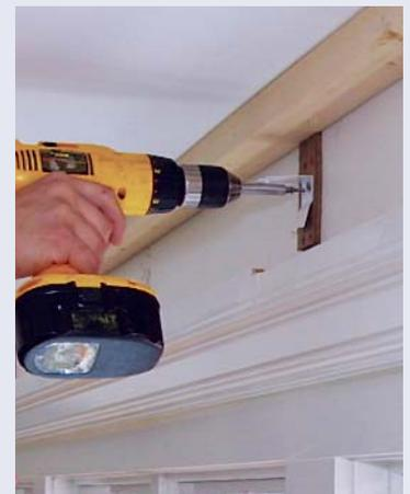
**2 Blocking guides the shade.** Mounting the hardware on ¼-in. blocking pushes the shade away from the wall to prevent it from hanging up on the casing.
