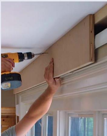
**3** **Screws fasten MDF to the cleat.** Countersunk and filled, trim screws offer the strongest hold on the weighty MDF. Biscuits align pieces of MDF to form the 18-ft. face of the valance.
