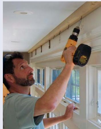
**1 A cleat supports the valance.** Screwed into the ceiling, the 2x3 creates enough space off the wall to house the shade and offers blocking for the face of the valance.
