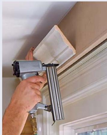
**4** **Crown molding adds a nook for lights.** Visually tying the valance into its surroundings, 4 $\frac{3}{4}$ -in. crown molding also creates a place to hide fluorescent lights.
