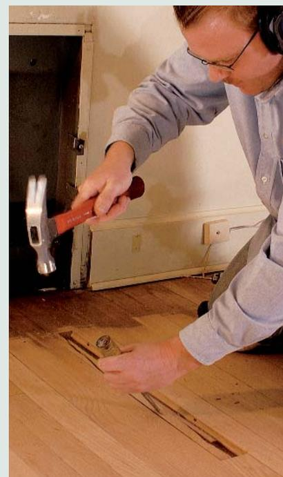
Use a chisel to remove the pieces of the old board. Always remove the pieces working away from the good floorboards.
