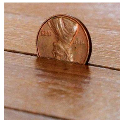
**If it's safe to drive, it's safe to sand.** The penny gauge for tire-tread wear works for tongue-and-groove floorboards, too. If you can cover part of Lincoln's head, there's enough wear layer for another sanding.
