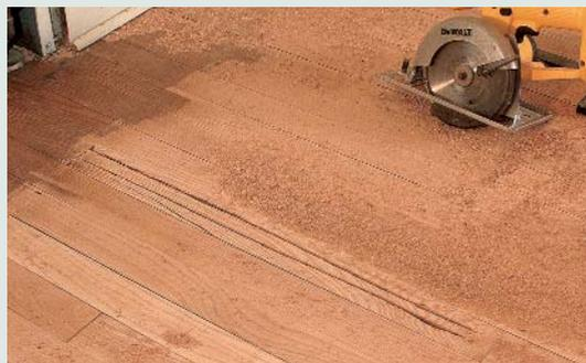
With a circular saw, make two cuts down the length of the board.
