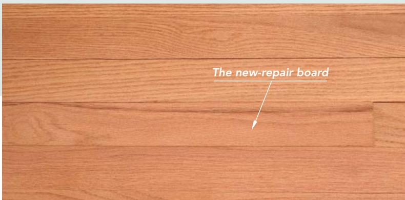
After the replacement is glued and nailed, nail holes and board edges are patched, then sanded. The replacement blends perfectly.
