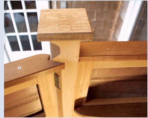
Simple joinery, yet elegant joints. The ipé cap of the shower doors embraces a cedar post. Saw kerfs in the cedar frame hold the copper panels in place.
