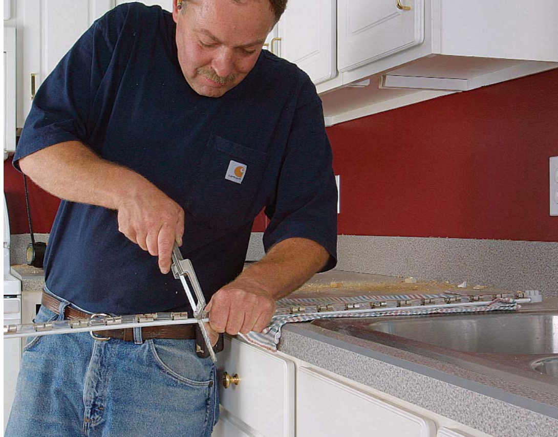
The plastic track is cut easily. After removing a bulb, cut the track 2 in. short of the cabinet length with a hacksaw. Holding the light track 1 in. short of the cabinet sides avoids a bright glare at the end of cabinet runs.
