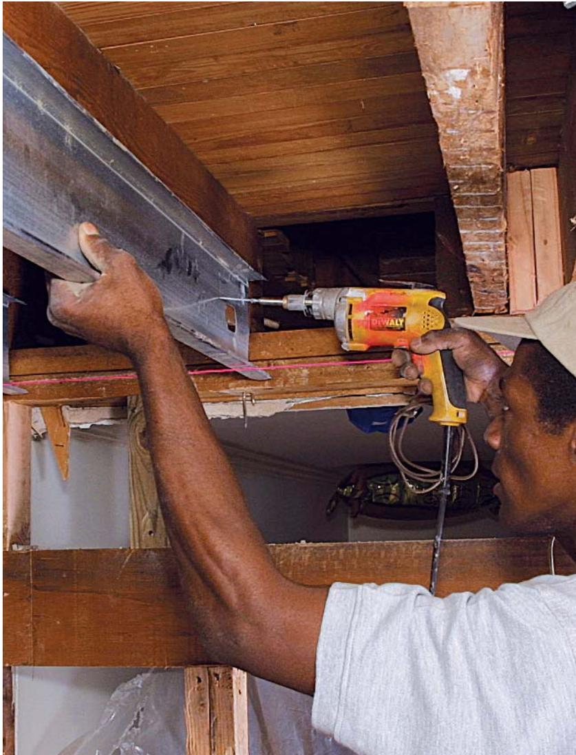
If wires or pipes run across the bottom of the joists, notch the studs around them (photo right). Where blocking requires notching the top of the stud, it sometimes makes sense to cut off the top flange altogether (photo far right).
