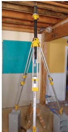
Laser levels and tripods are available at most rental centers. A water level also could have been used on this project. A bubble (or spirit) level, however, would have been awkward and unreliable for this type of project, unless the room had been small.
