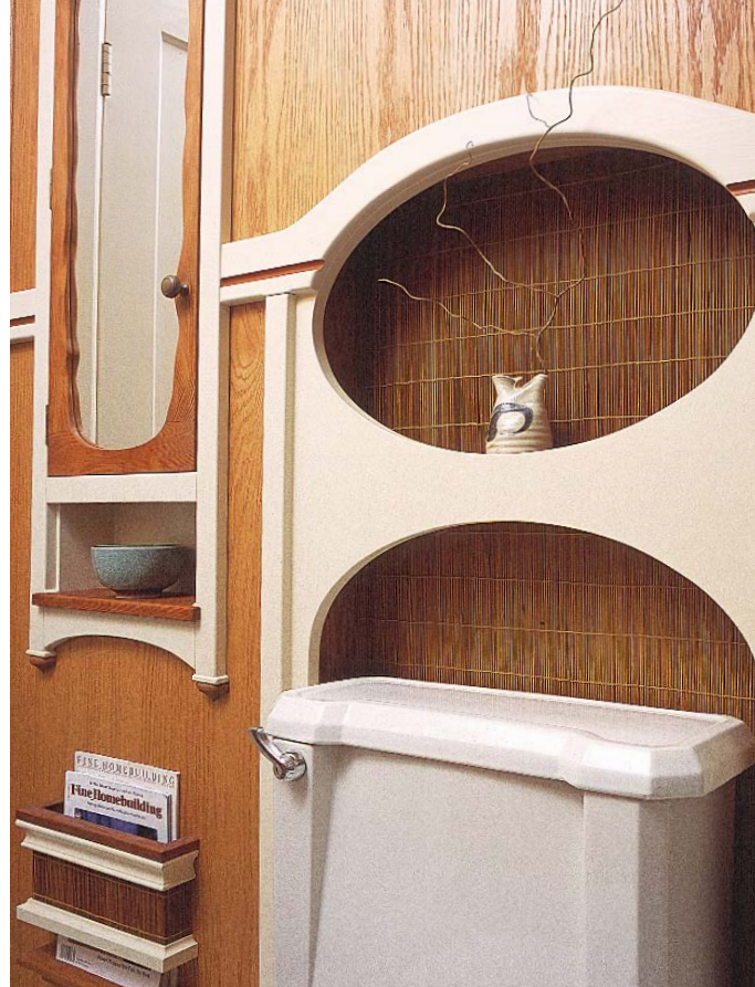
Take advantage of the space between the studs. Oregon builder Gordon Kadar saved some precious floor space by recessing his toilet's tank into the wall (photo above). The HY-DIT cabinet (photo left) provides compact storage for maintenance supplies (970-523-6935; www.hy-dit.com ).
