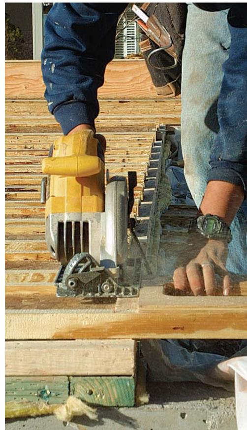
**After aligning the joists, snap a chalkline and cut them to length in place. Beware of anchor bolts lurking below when making this cut.**
