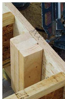
Bearing (or squash) blocks are installed at all point loads. But to avoid confusion with other layout marks, they aren't located and installed until after the rim joist is in place.
