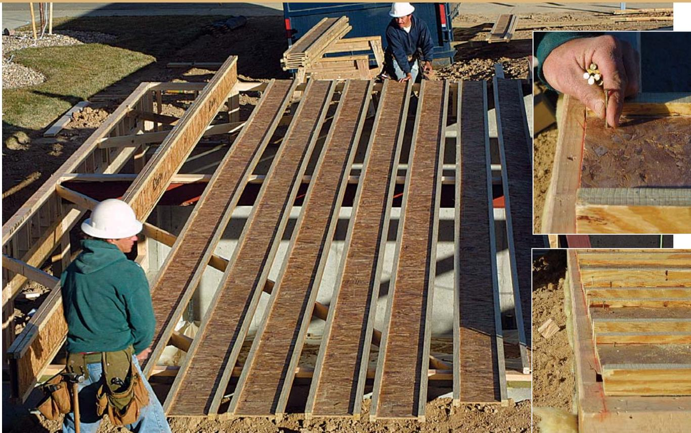
**Position the square ends of each joist to the chalkline (the rim-joist line) and tack them into place along their 16-in. o.c. layout lines. Later, the 8d nail will act as a hinge when the joists are stood upright.**
