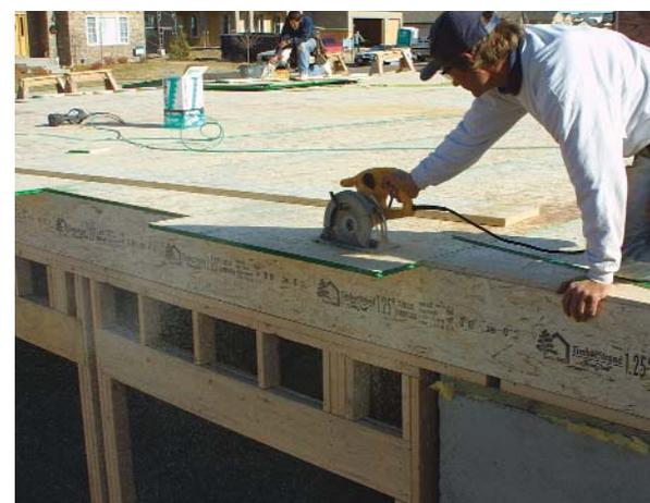
**Cut the sheathing in place. Run sheets long at the ends, snap a chalkline, and cut off the excess. This process is faster and turns out a better floor than cutting each piece to fit.**
