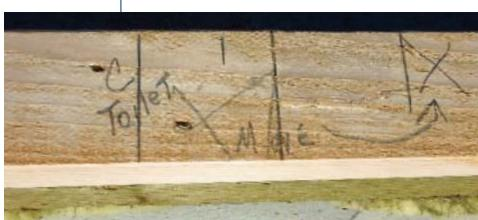
If the last joist bay is less than 12 in., make it a full 16 in. to allow plumbers, HVAC, and electricians more room.
