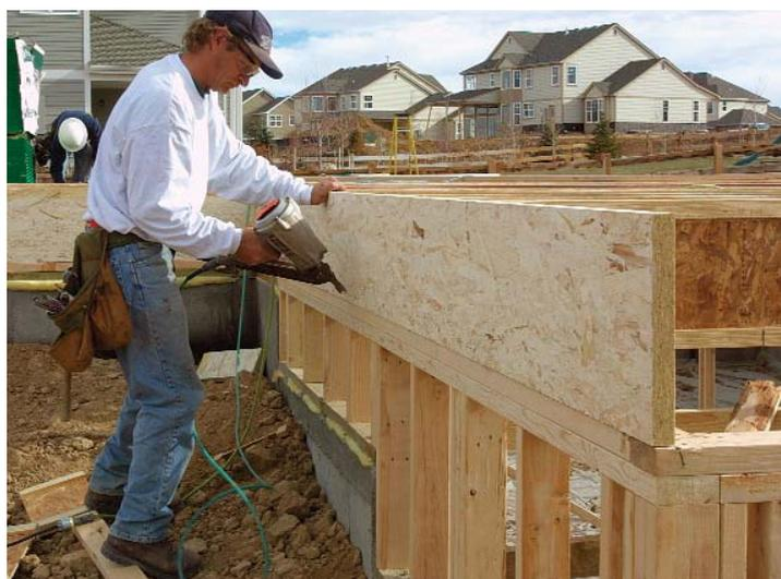
“...We start from one end of the house, roll the joists, and nail them in place ... we usually can stand the joists for 40 lin. ft. of floor in about 10 minutes.”
