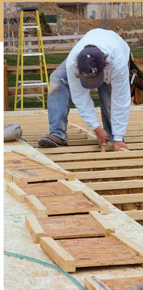
**Sheathe your way over to where blocking is needed. Do not walk across unstable joists or work from a ladder below the floor. Sheathe over to the beam, then add the joist blocking.**
