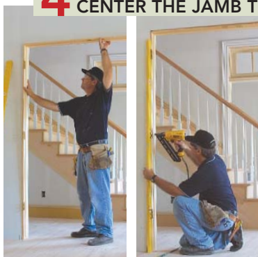
Set the jamb along the shimmed trimmer first.
