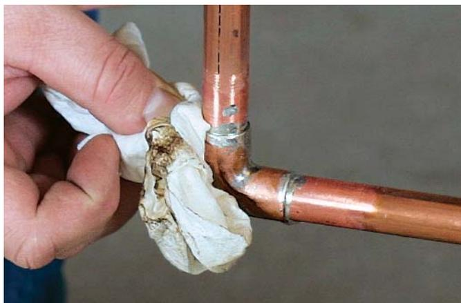
**10** **Not just for show.** Even if the pipe is to be buried beneath drywall, always wipe the solder with a rag before it has had time to cool. A bright, uniform solder joint between the fitting and the pipe is proof of a job well done.
