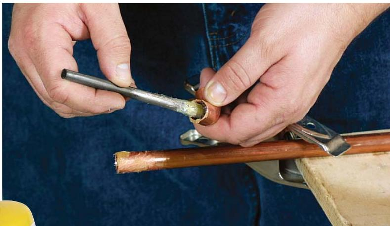
**6 Apply flux to deep-clean the metal.** Brush a liberal coating of flux onto both surfaces (the flux removes minute traces of tarnish and etches the copper to promote adhesion with solder). To prevent contaminating the flux, close the cover tightly when not in use, and store the brush in a plastic bag.
