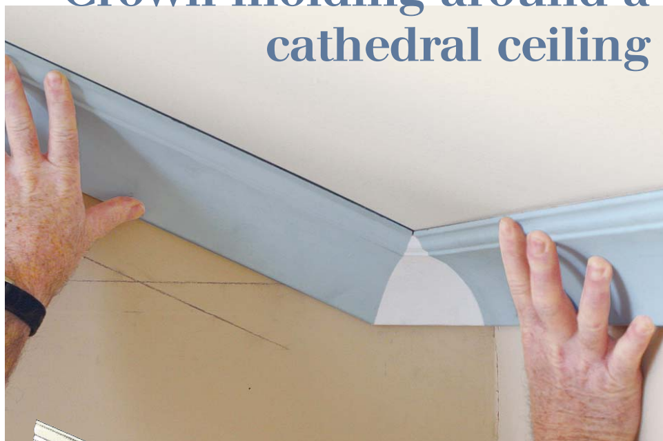
The problem and the solution. When crown molding runs up a vaulted ceiling, the profiles won't match at the corner (drawing left). So instead of using different-size moldings, a transition piece turns the corner using the same profile (photo above).
