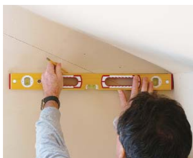
Draw a level line from the corner.
