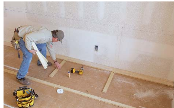
The writing is on the wall. A full-size layout on the wall lets the author see the wainscot's proportions and serves as a guide for assembly.
