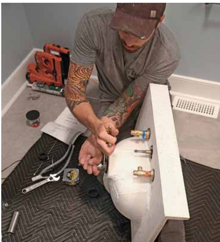
Easy access. It's much easier to install and align the faucet before setting the countertop than it is to reach underneath after it's installed.
