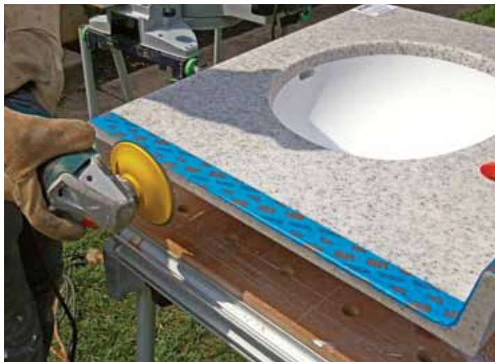
Sand to fit. Solid-surface counters can be cut and shaped with carbide tools and then sanded down to a scribe line using an angle grinder equipped with a sanding disk.
