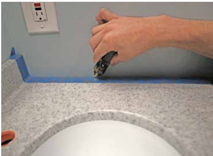
Get a good mark. A strip of painters tape makes a pencil-friendly path for marking hard, glossy countertops with a scribe tool.
