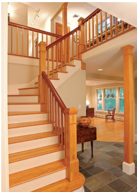
The well-lighted stairwell. Built in the location of the original attic stairs, the new staircase brings light into the center of the house. Photo taken at C on floor plan.
