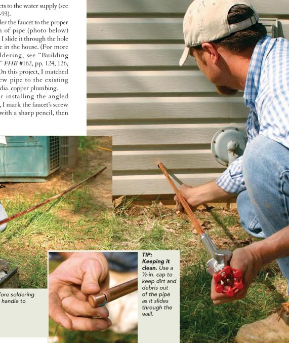
Open the handle, and solder the joint. Before soldering the faucet to the new copper pipe, turn the handle to prevent the seat from melting.
