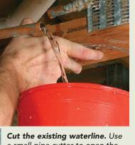
**Cut the existing waterline.** Use a small pipe cutter to open the old pipe to prepare for the new joint. After opening the downstream faucet, pull the existing pipes down slightly to drain the remaining water.
