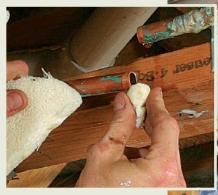
TIP: A ball of white bread shoved into the pipe temporarily blocks water flow while the pipe is being soldered. But you need to move fast to solder the joint before the bread dissolves.
