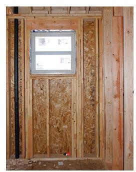
Most framers think structurally, not thermally. This photo was taken three miles down the road from the houses on the previous page. These massive thermal bridges and hard-to-insulate cavities will make this a frigid wall. Because it's a bathroom, a mold problem is likely.
