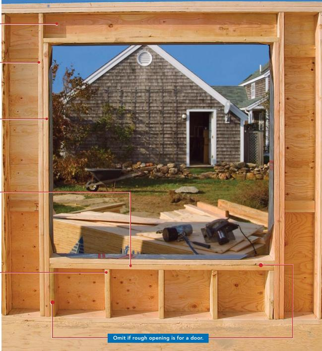
Ithough the name suggests otherwise, rough openings demand plenty of precision, especially when they are framed in load-bearing walls. Properly done, rough openings provide a place for windows and doors to fit securely, unaffected by the critical structural work being done by headers, king studs, trimmers, sills, and cripples (or sill jacks). After years of building, I've learned that getting rough openings right makes the rest of the job go smoothly.
