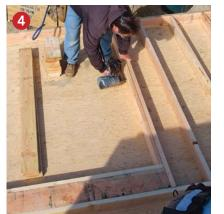
studs on each side of the header should be straight in all directions (for example, no bow, crown, or twist). The header needs to be sized appropriately and should provide room for insulation, if possible.
