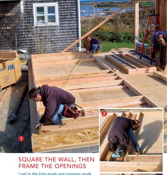
I nail in the king studs and common studs first, leaving out any commons that will get in my way later when I'm nailing in the header. 1 Then I square up the wall and tack it to the deck to keep it that way while I finish the rough openings. 2 I install the header between the king studs next, 3 then nail in any commons that were left out.
