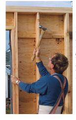
Final detail. Once the wall is raised and braced, I finish nailing off the parts of the header that were not accessible while the wall was lying on the deck.
