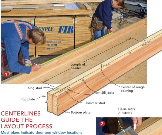
Most plans indicate door and window locations by noting a dimension to the centerline, so I start my layout by marking the centerlines on the wall plates. 1 Then I measure half the width of the rough opening on both sides of the centerline. 2 Using a Speed Square, I finish marking the trimmer and king-stud locations.
