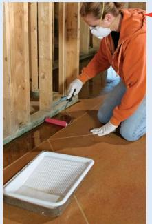
1. Sealers can be used to protect an entire floor. Here, though, an oil-based sealer is rolled on only around the border for a decorative effect.
