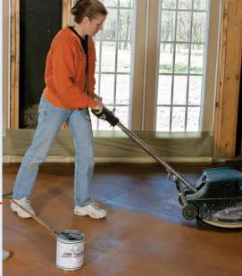
**2.** After the sealer has dried, apply a stand-alone paste wax with a rotary floor machine and a stiff natural-bristle brush. Finish by polishing the floor with a soft white polishing pad (photo p. 83).
