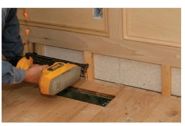
Add blocking at stud locations to support the baseboard. Only a small part of the baseboard will overlap the bottom of the panel, so this backing provides nailing blocks for the baseboard.
