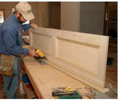
Add the apron now to save your knees. While the panel is upside down on the workbench, attach the apron molding and apron returns. Remember to run each return past the back of the frame 1/4 in. so that it will meet the wall when it's installed.
