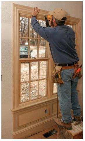
Install the head casing last. Nail the legs of the casing on first, keeping the same reveal between the casing and the jamb that was used between the stool and the jamb. Cut the head casing to fit, finetuning the angle as needed for a tight miter joint.
