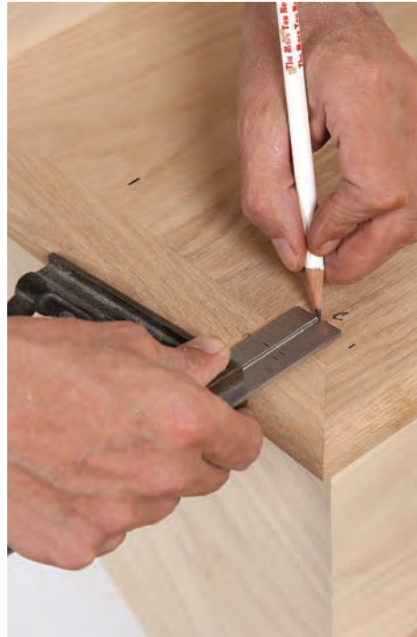
Center the placement. The vertical centers of the balusters should be aligned with the vertical centers of the newels, and are easy to locate consistently using a combination square referenced off the tread returns.
