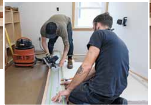
Rip the bevel on the top rail. Using the end stiles that are already fit to the ceiling as a reference, Young rips a bevel along the top rail with a track saw.
