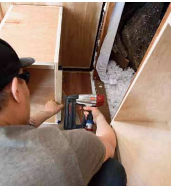
Blocking for height. Ripped to the necessary dimensions, blocking is nailed to the front and back edges of the carcasses' bottoms to set their heights above the finished floor.
