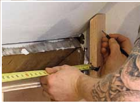
Measure for the rails. With the end stiles cut to length, scribed to the walls, and temporarily tacked in place, Young measures for the top and bottom rails.
