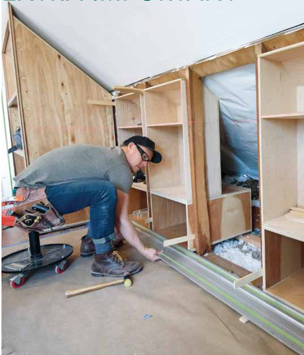
Blocking for height. Ripped to the necessary dimensions, blocking is nailed to the front and back edges of the carcasses' bottoms to set their heights above the finished floor.
