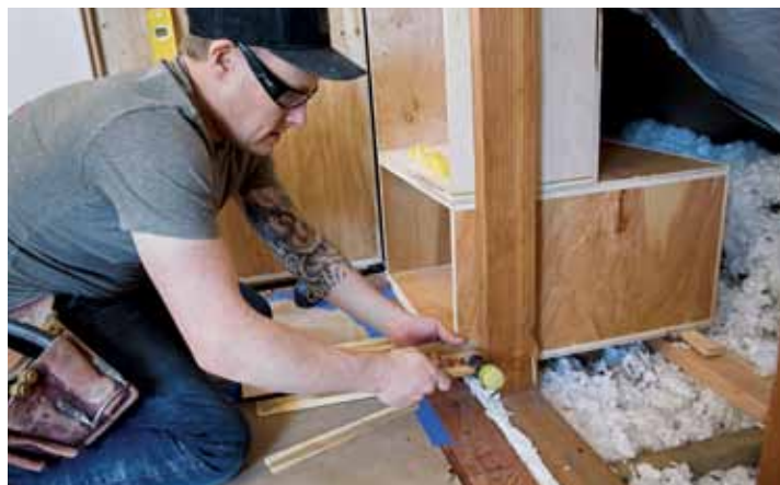
Ready, set, shim. Once each carcass is set plumb with shims beneath the back of the drawer boxes, more shims are used between the sides of the carcasses and the studs to ensure they stay square.
