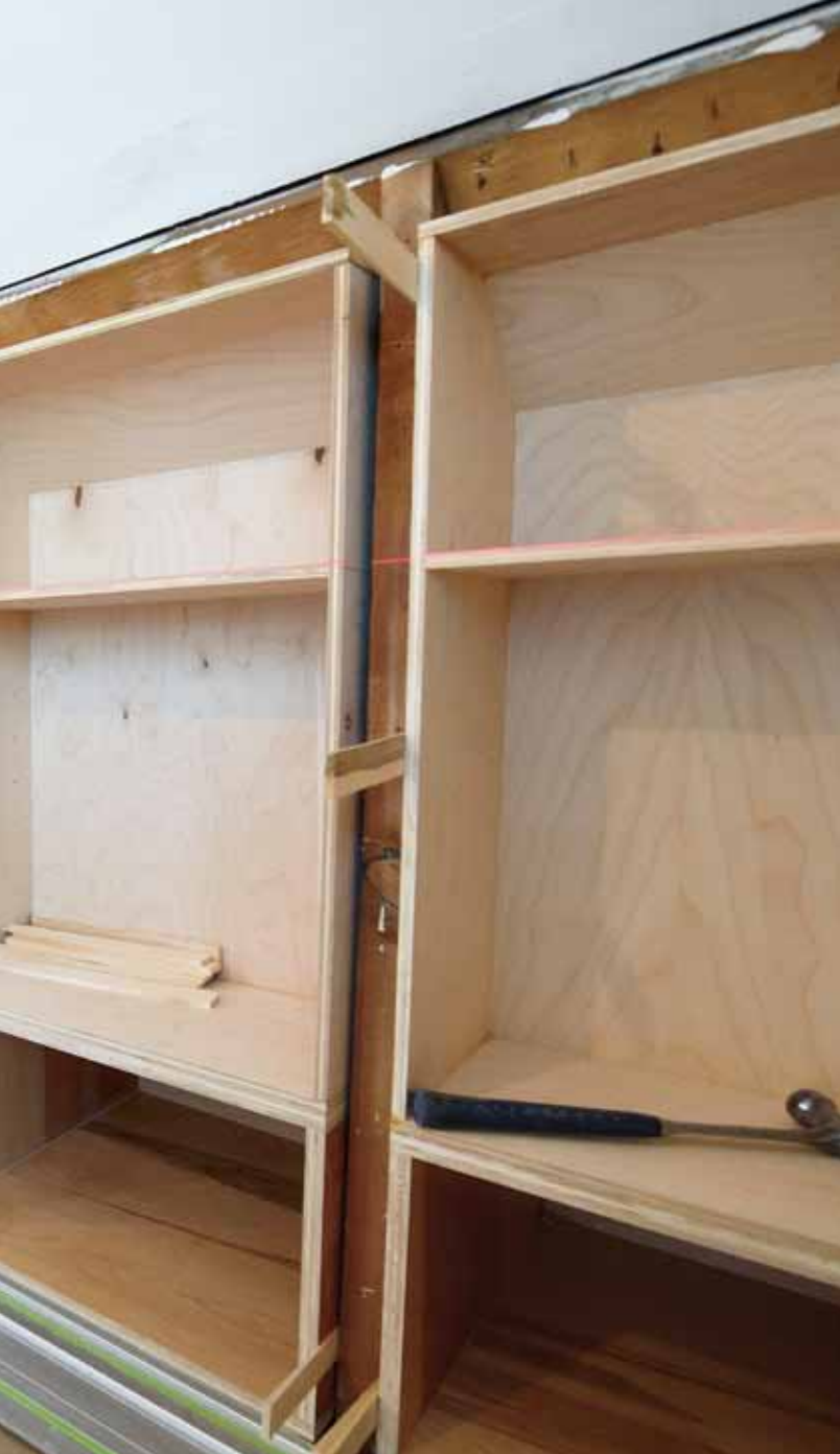
Ready, set, shim. Once each carcass is set plumb with shims beneath the back of the drawer boxes, more shims are used between the sides of the carcasses and the studs to ensure they stay square.
