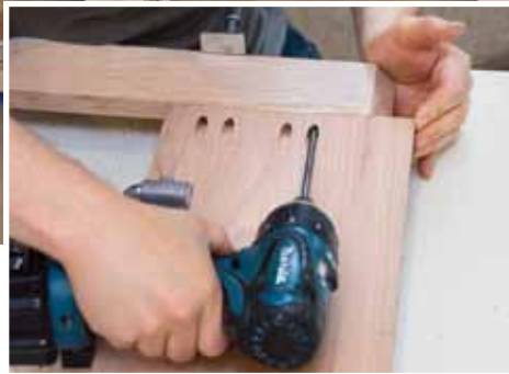
Assemble with pocket screws. The bottom and top rails are then fastened to the stiles with glue and pocket screws. The top rail is left wide to be scribed to the ceiling.
