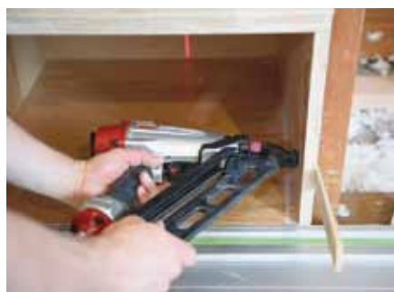
Ready, set, shim. Once each carcass is set plumb with shims beneath the back of the drawer boxes, more shims are used between the sides of the carcasses and the studs to ensure they stay square.
