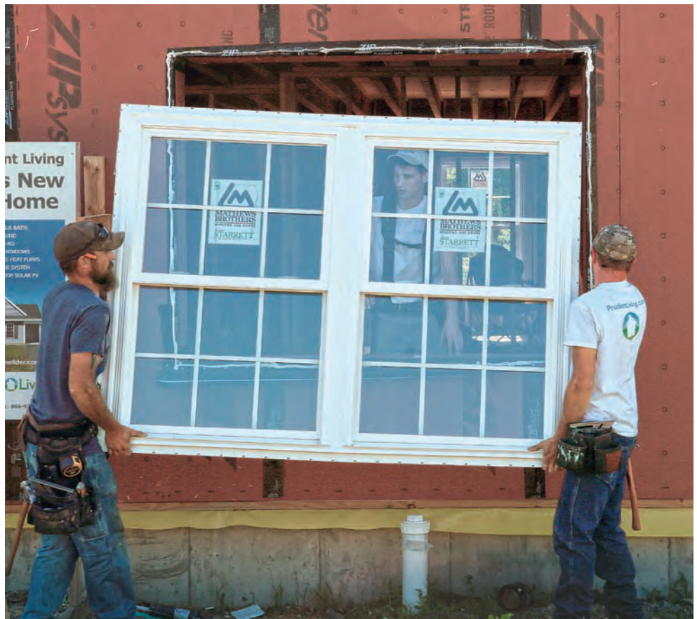
Zip System flashing. The window openings are flashed with a combination of Zip System standard flashing tape and their new stretch tape. The stretch tape makes a smooth transition through the corners so that the window flanges sit flat on the wall.
