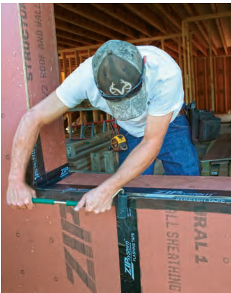
Zip System flashing. The window openings are flashed with a combination of Zip System standard flashing tape and their new stretch tape. The stretch tape makes a smooth transition through the corners so that the window flanges sit flat on the wall.
