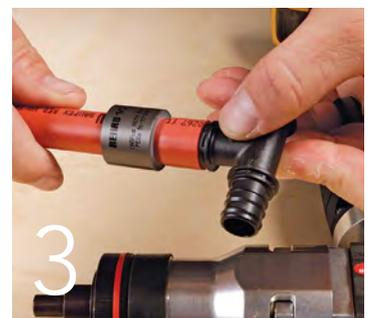
3 Remove the tool and immediately insert the fitting so that the tubing is snug against the fitting's stop.
