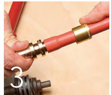
3 Release and remove the expansion tool, and immediately insert the fitting so that its last barb is just shy of the end of the tubing (about 1/16 in. away).
