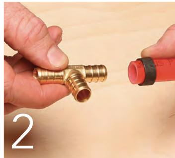
2 Align the crimp ring so that it's about 1/8 in. to 1/4 in. from the end of the tubing. Aim to have the ring aligned over the fitting's central ribs.
