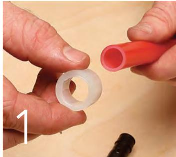
1 Slide a ProPEX ring over the end of the tubing. Insert the tool head into the tubing, and expand the tubing and sleeve.
