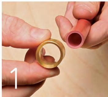
1 Slide a compression sleeve onto the tubing, beveled end toward the fitting, pushing it far enough so it won't interfere with the expansion process.
