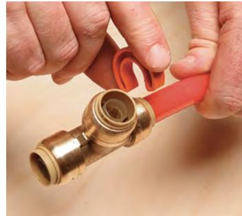
To remove the fitting, place the removal tool over the tubing, and press it against the fitting's plastic collar until the fitting releases.
