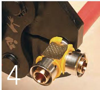
4 Squeeze the trigger to engage the tool and press the fitting.
