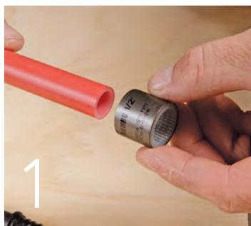
1 Slip a sleeve onto the tubing, sliding it back far enough that it doesn't interfere with the expansion.
