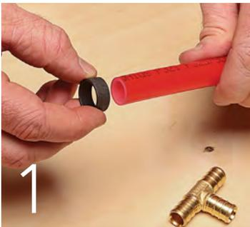
1 Slide a copper crimp ring onto the tubing, then insert the fitting into the tubing, making sure it's fully seated.
