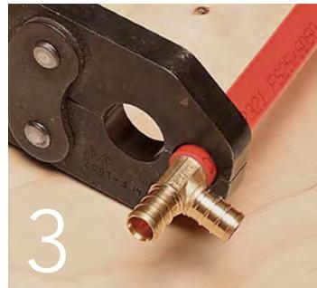
3 Fit the crimp tool's jaws over the ring and squeeze the handles all the way to crimp the ring into place.
