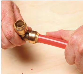
Slide the fitting onto the tubing until it bottoms out.
