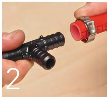
2 Insert the fitting into the tubing, making sure it's fully seated.
