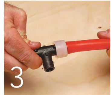
3 Remove the tool and insert the fitting so its shoulder is snug against the sleeve. The fitting should be secure within seconds.
