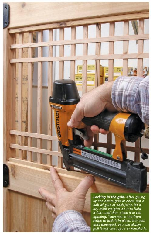
on both sides of it, like glass stops. If the gridwork ever gets damaged, it will be a cinch to pop it out and repair or replace it.
