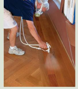
**Apply a thin, even coat.** You can apply the shellac with a brush or synthetic pad, but I prefer to spray it on because spraying is faster than other methods. Whatever technique you use, don't apply a thick coat. The sealer dries fast, so work quickly and maintain a wet edge. Depending on humidity level and temperature, the floor will be ready to sand in two to three hours.
