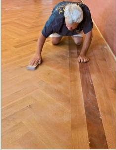
Sorry, but hand-sanding works best. The purpose here is to scuff-sand the sealer to a dull finish. I do this by hand because I am less likely to penetrate either of the preceding layers. Although 220-grit sandpaper does the job, fine sanding sponges work better because they don't clog as easily. Vacuum the floor completely after sanding.
