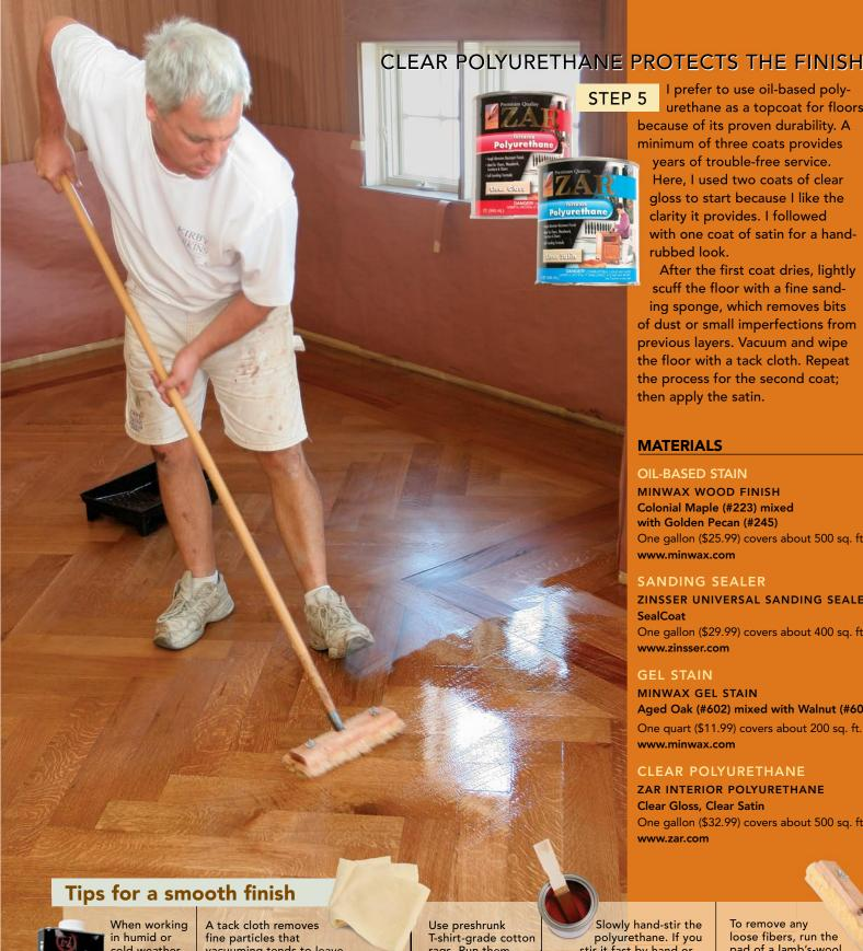
I prefer to use oil-based polyurethane as a topcoat for floors because of its proven durability. A minimum of three coats provides years of trouble-free service. Here, I used two coats of clear gloss to start because I like the clarity it provides. I followed with one coat of satin for a hand-
