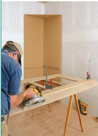
The sides of the face frame are cut at a 47° bevel. This makes for a snug fit against the wall and the front of the carcase. For this hutch, I used an 8-in. border on the sides of the face frame. Anything smaller starts to compromise the strength, and anything larger looks clunky and awkward.
