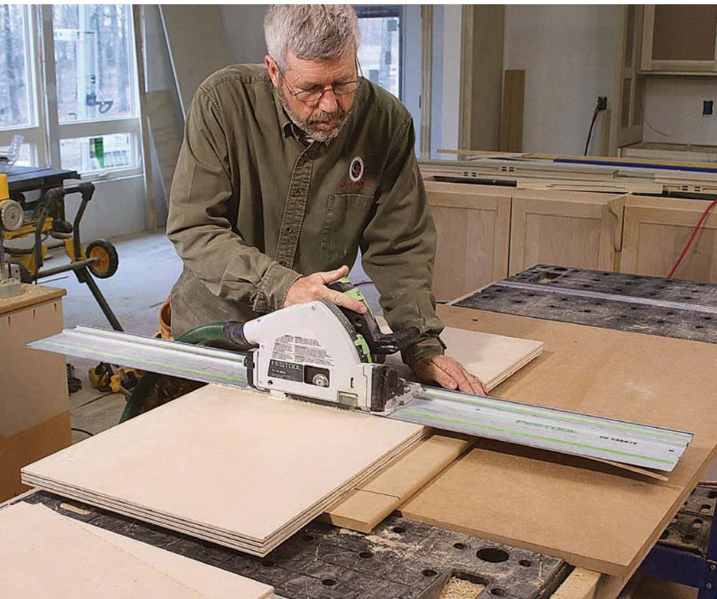
**Perfect panels.** A track saw makes quick work of breaking down the  $\frac{1}{2}$ -in. plywood sheets used to make the door panels. Clip all four corners of each panel on the miter saw for an easy fit during glue up.
